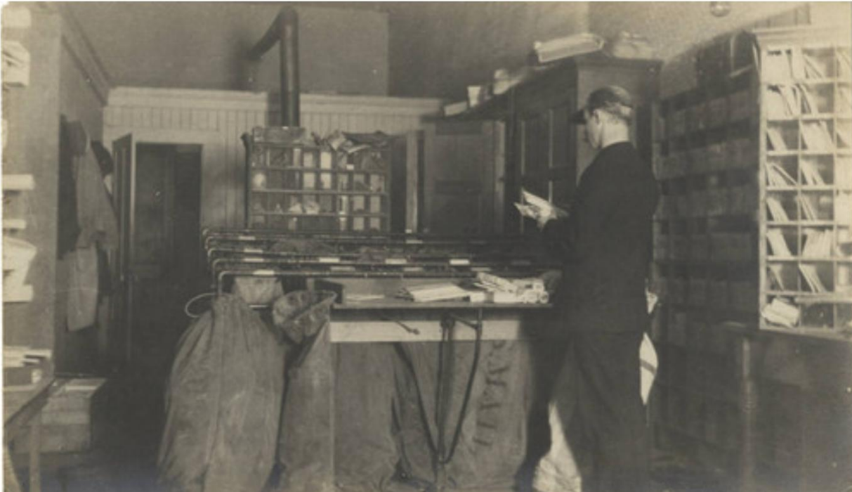
Two pictures of the inside of the Post Office ca 1905
